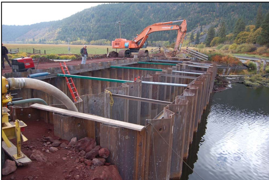
Figure 9-11. Photo of Fish screen/irrigation diversion under construction at Running Y Ranch, October 2009.
